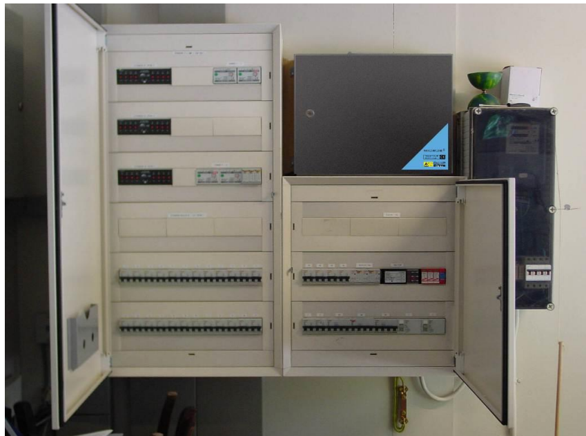
Figure 1: MICROS+ outside distribution board
